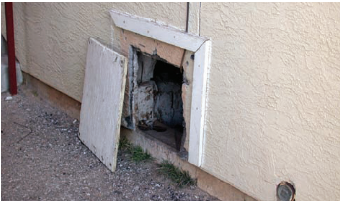
Access panels should not be left open
