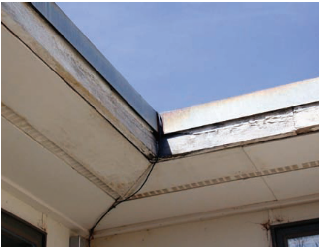
Openings under roof line
