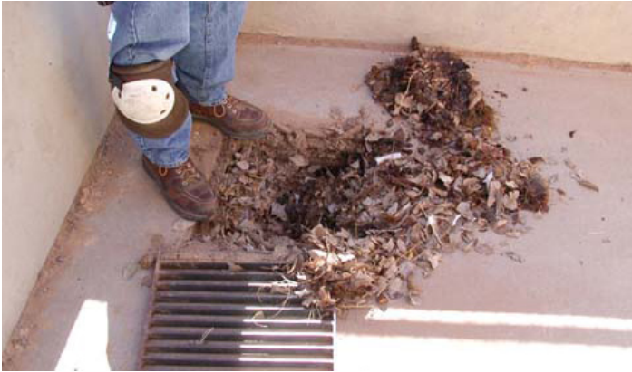
Grate and drain covers should be removed and cleaned out periodically
