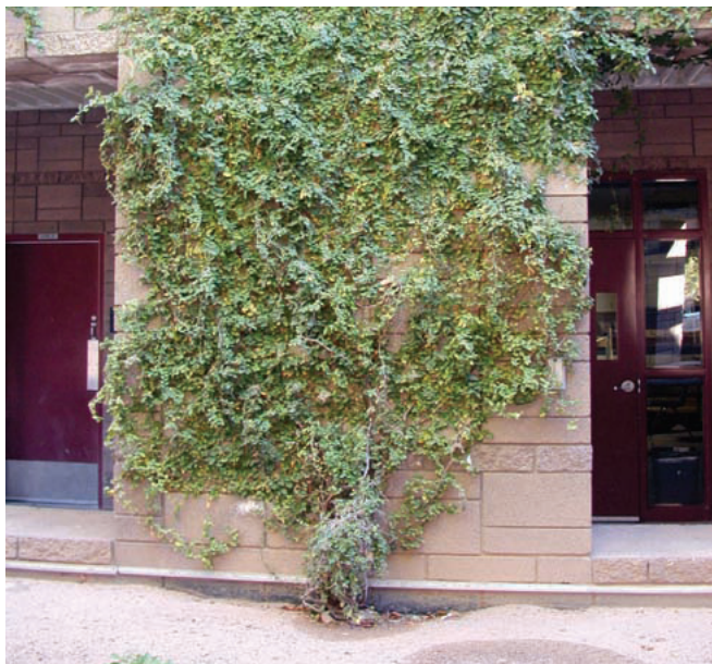
Vine against the wall provides pest harborage areas and access to the building
