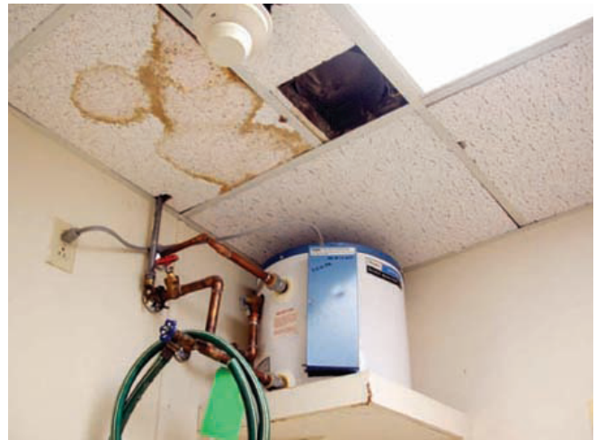
Tiles in drop ceiling indicating a plumbing leak
